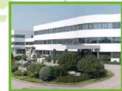
Suzhou Sodick Special Equipment Co., Ltd.
