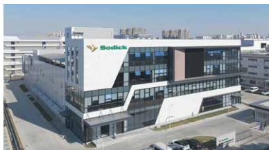
7 Suzhou Sodick Special Equipment Co., Ltd.
