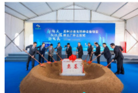
Construction of the New Suzhou base begins (Scheduled to start operations in September)
