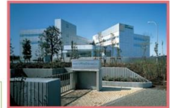
Head Office/Research and Technology Center
