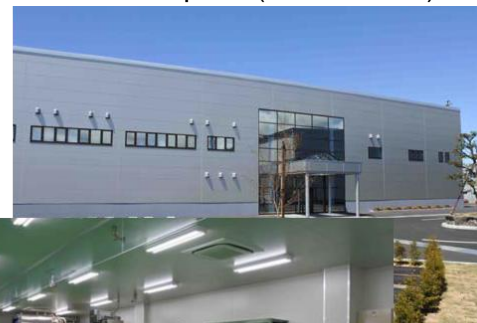
➤ The new plant (outside view)
