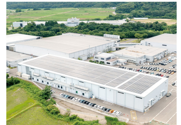
Kaga Office's newly installed solar power generation system
