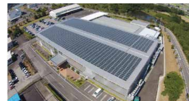
▲ The rooftop solar power array at the Sodick F.T. Miyazaki Office
