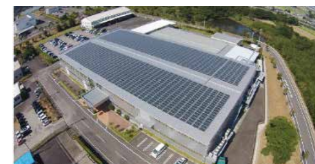
▲ The rooftop solar power array at the Sodick F.T. Miyazaki Office
