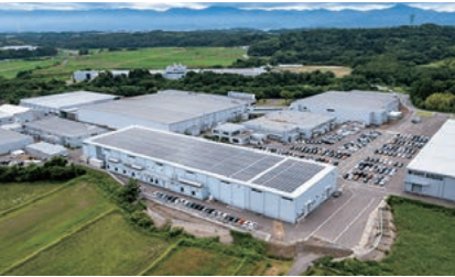
The rooftop solar power array at Kaga Factory
