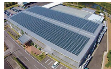
The rooftop solar power array at the Sodick F.T Miyazaki Factory
