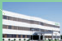
Suzhou Sodick Special Equipment Co., Ltd.
